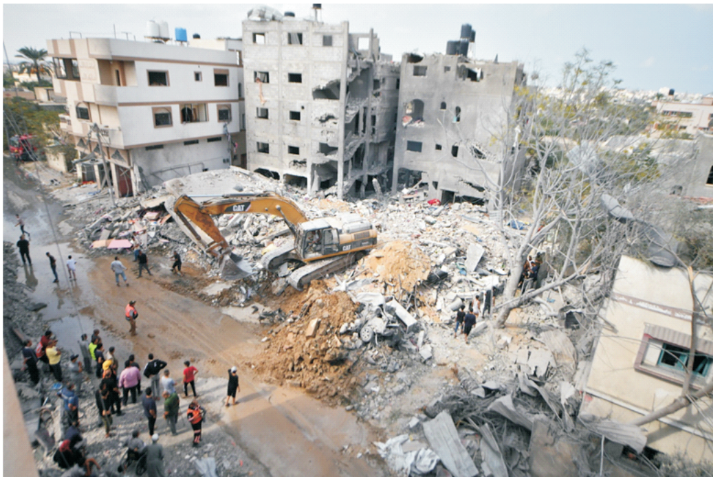
Plate 2: Depict the destruction of building
