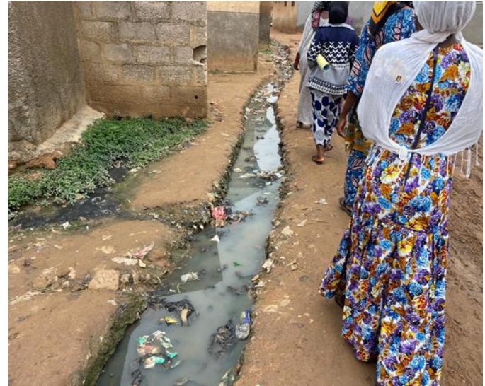
Plate 4: A clogged drainage,
